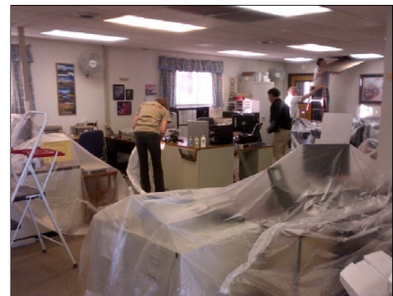
IFMA volunteers replacing ceiling tiles at the Denver Rescue Mission
